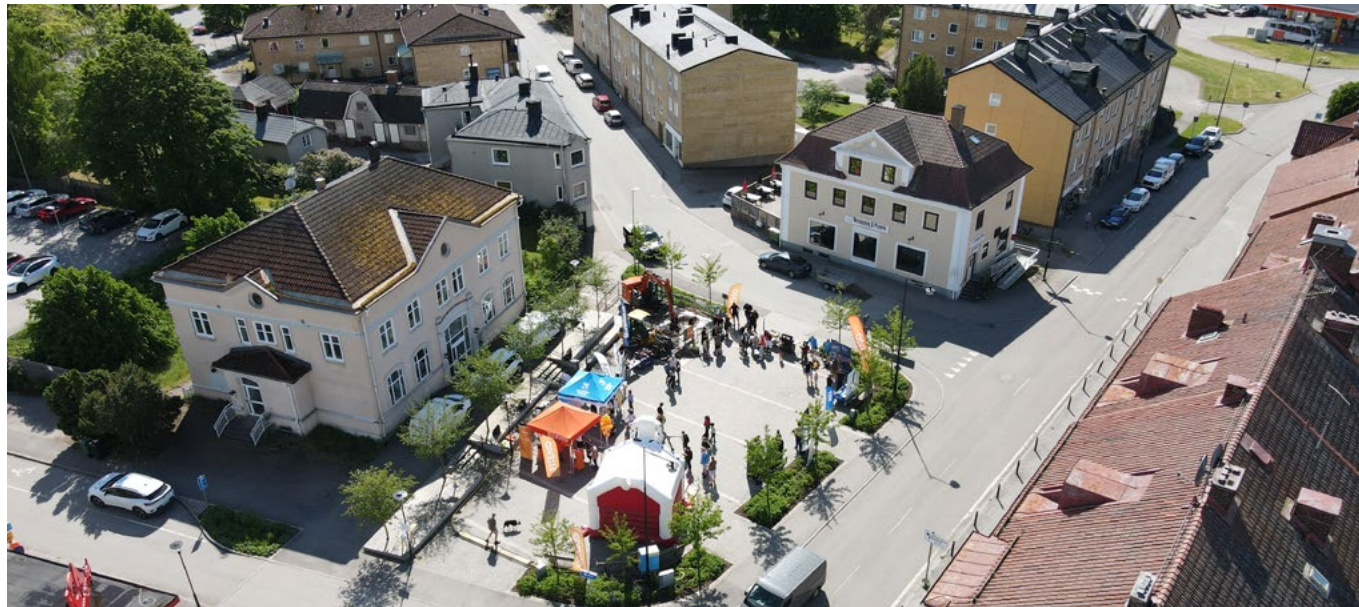
In Gullspång Ellevio built two new substations and seven kilometres of underground cable in 2024. The cable project was entirely powered by electricity.
