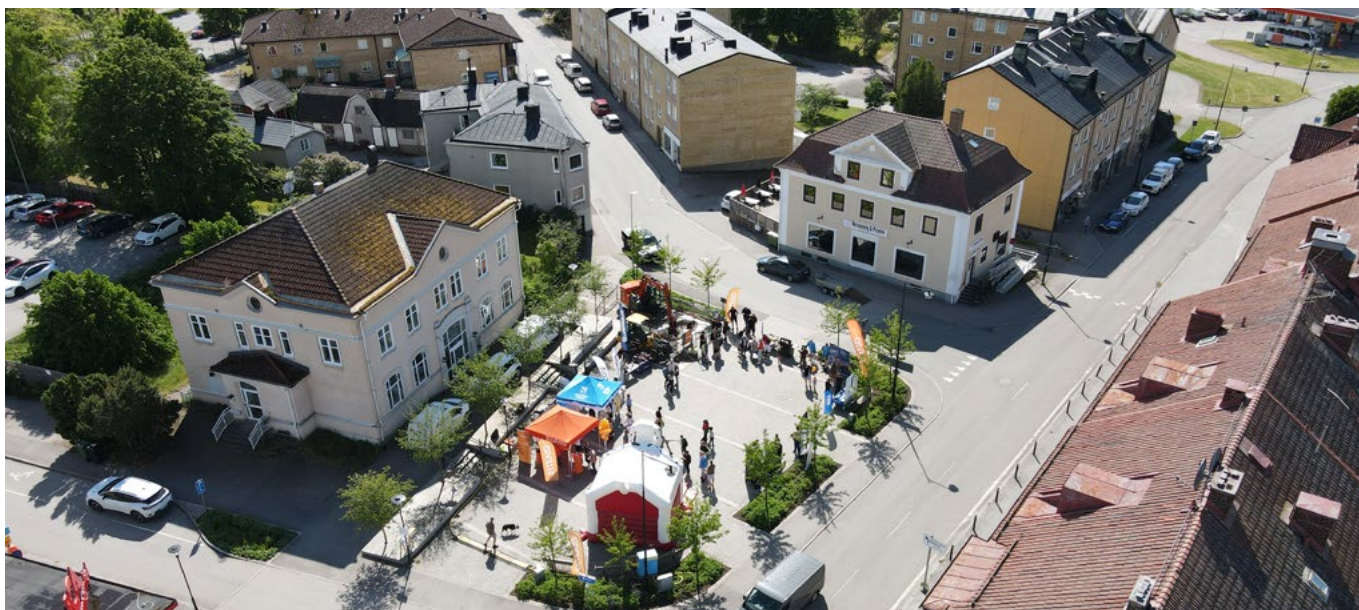
In Gullspång Ellevio built two new substations and seven kilometres of underground cable in 2024. The cable project was entirely powered by electricity.
